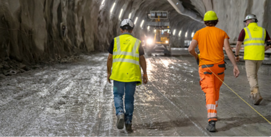
Tunnel in der Aushubphase © GIF Photos
